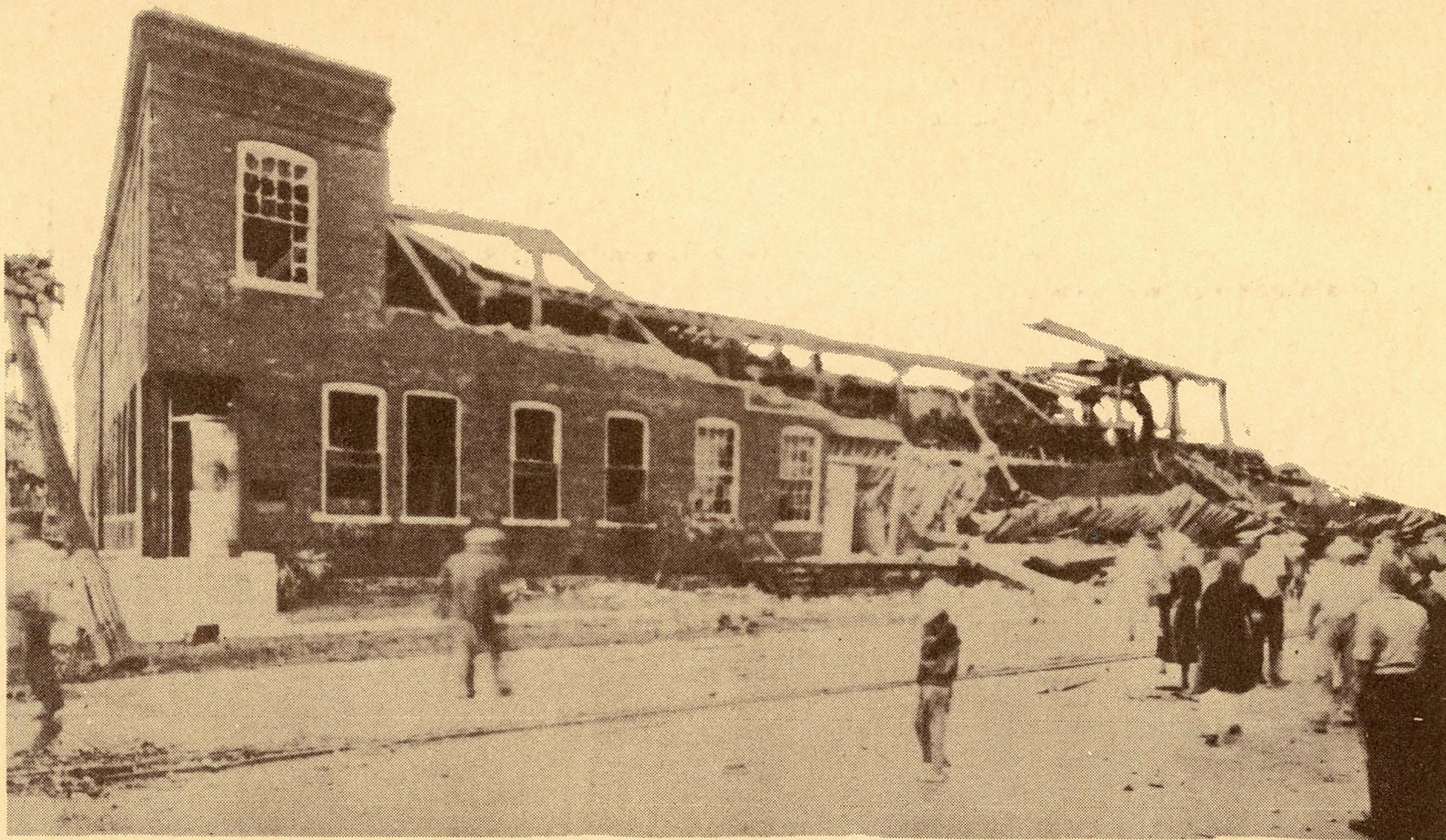
ELCO TOOL CO, PLANT ON BROADWAY IN RUINS, ROCKFORD TORNADO.
