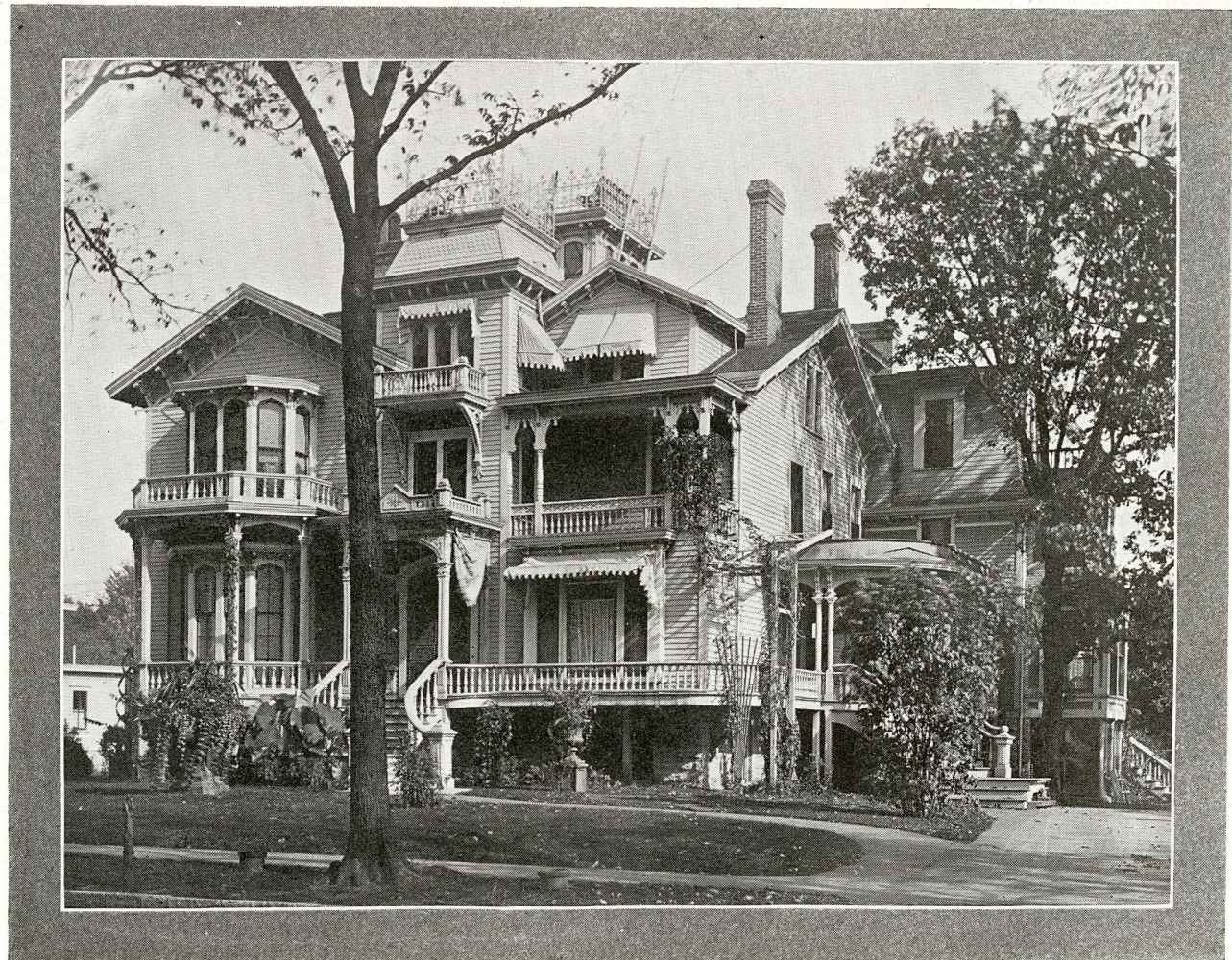
RESIDENCE OF RALPH EMERSON
