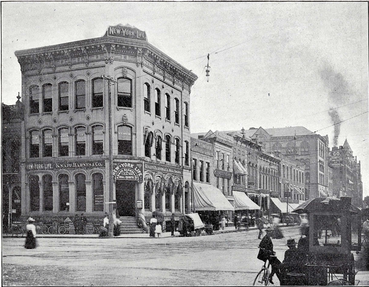
MAIN STREET, Looking South.
