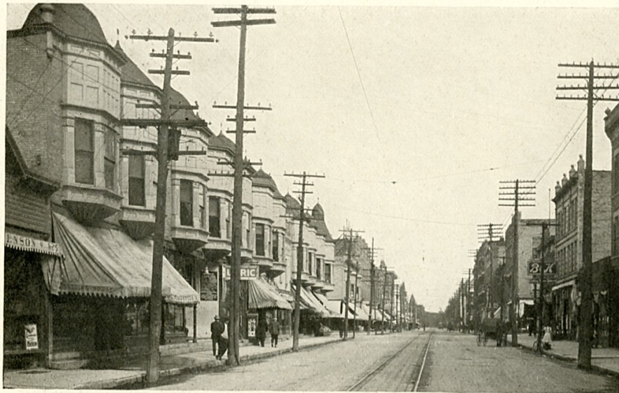
SEVENTH STREET—LOOKING NORTH
