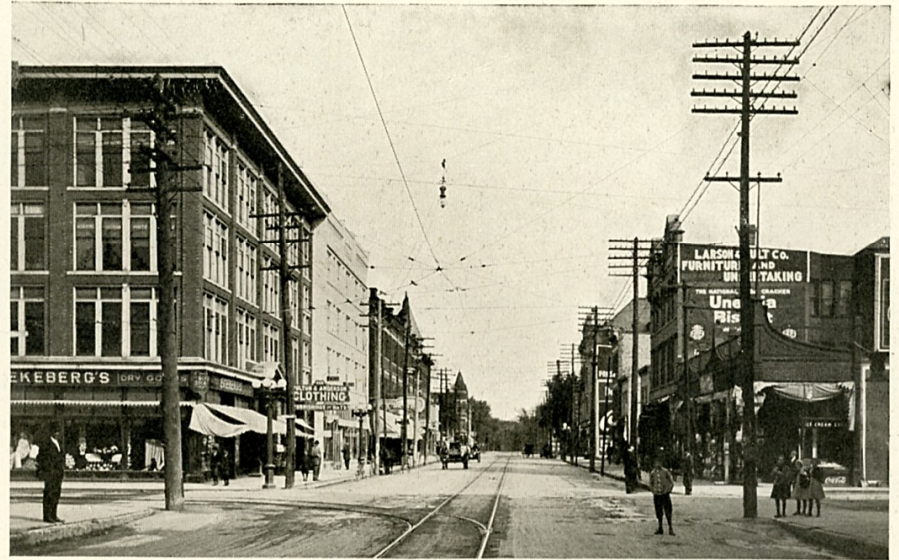
SEVENTH STREET—LOOKING NORTH
