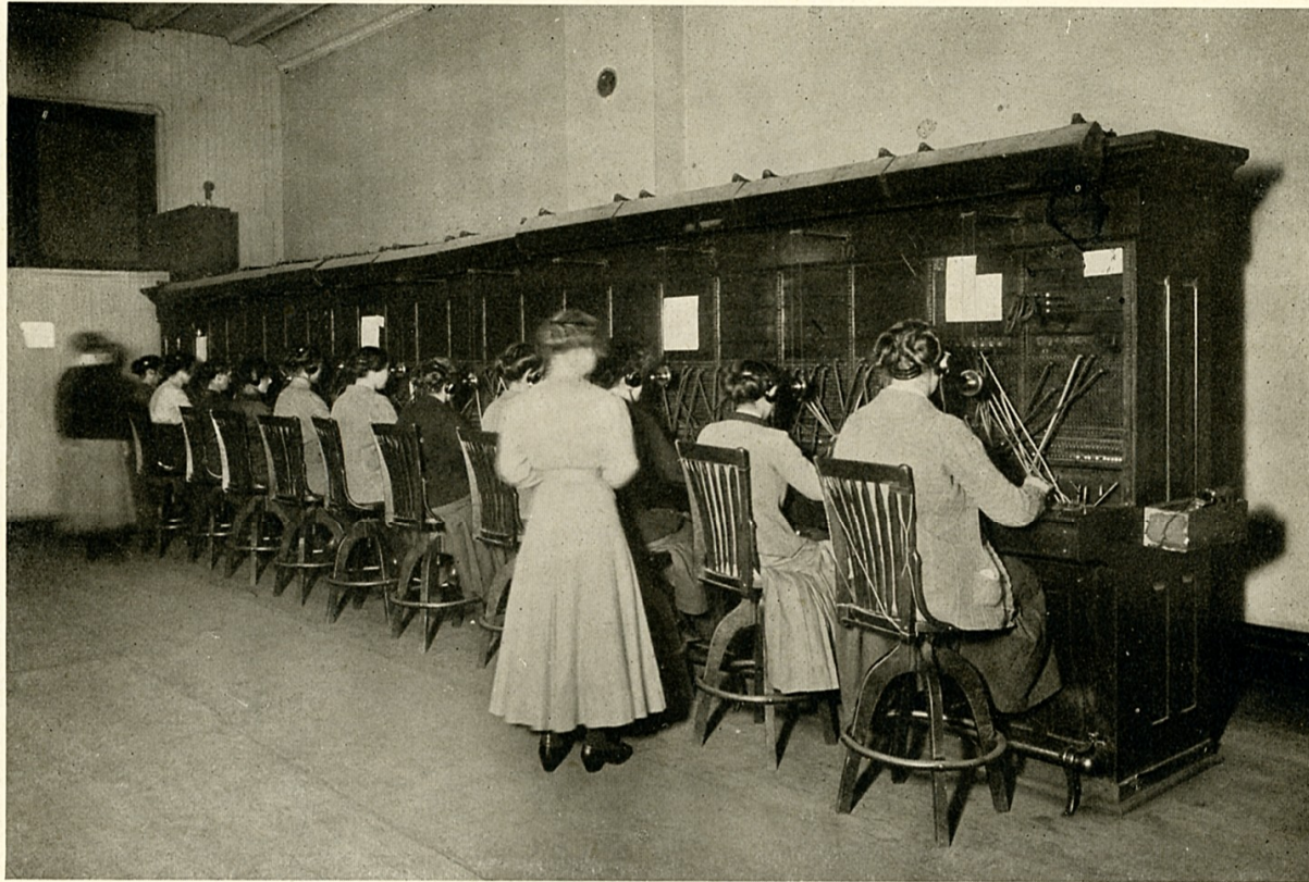
ROCKFORD HOME TELEPHONE CO.—PART OF OPERATING ROOMS
