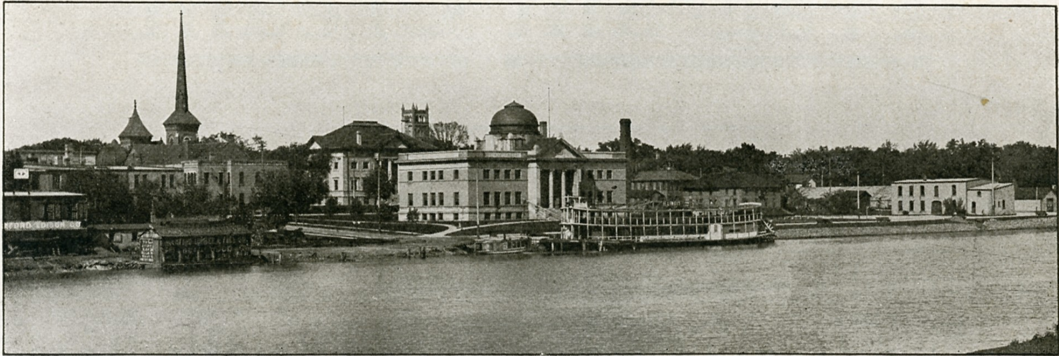
WATER WORKS FRONT
