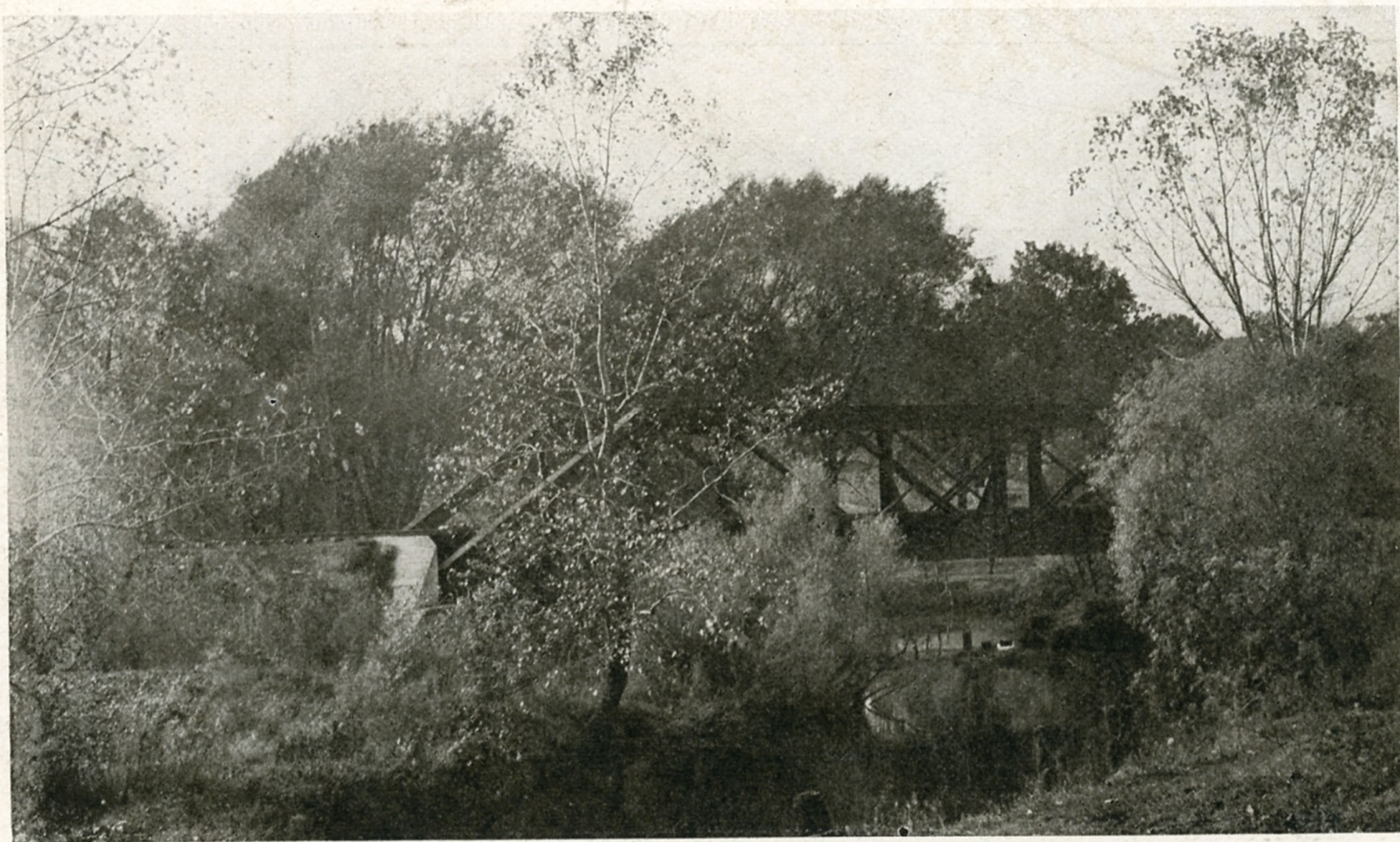
C. M. & ST. PAUL RAILROAD BRIDGE OVER KENT CREEK
