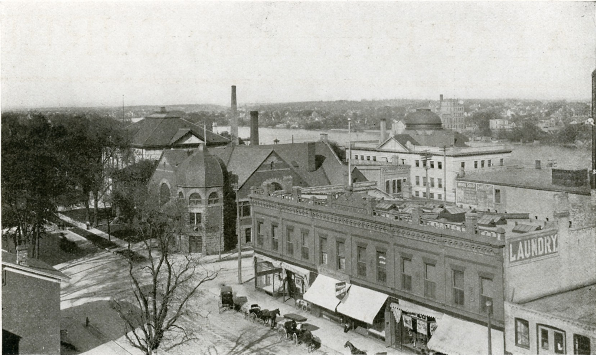
VIEW ON NORTH MAIN STREET
