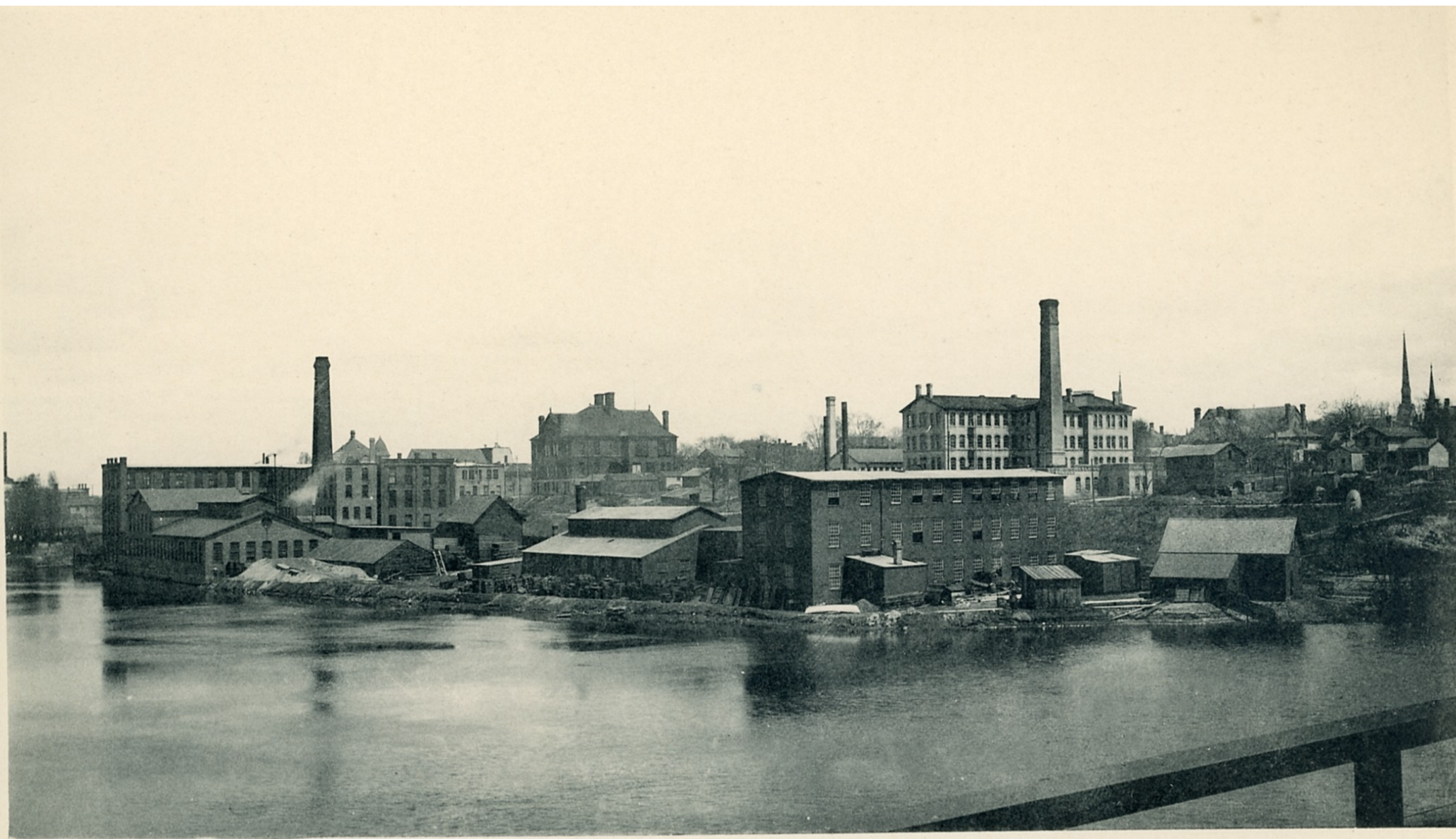
VIEW ON EAST BANK OF ROCK RIVER LOOKING NORTH FROM RAILROAD BRIDGE.
