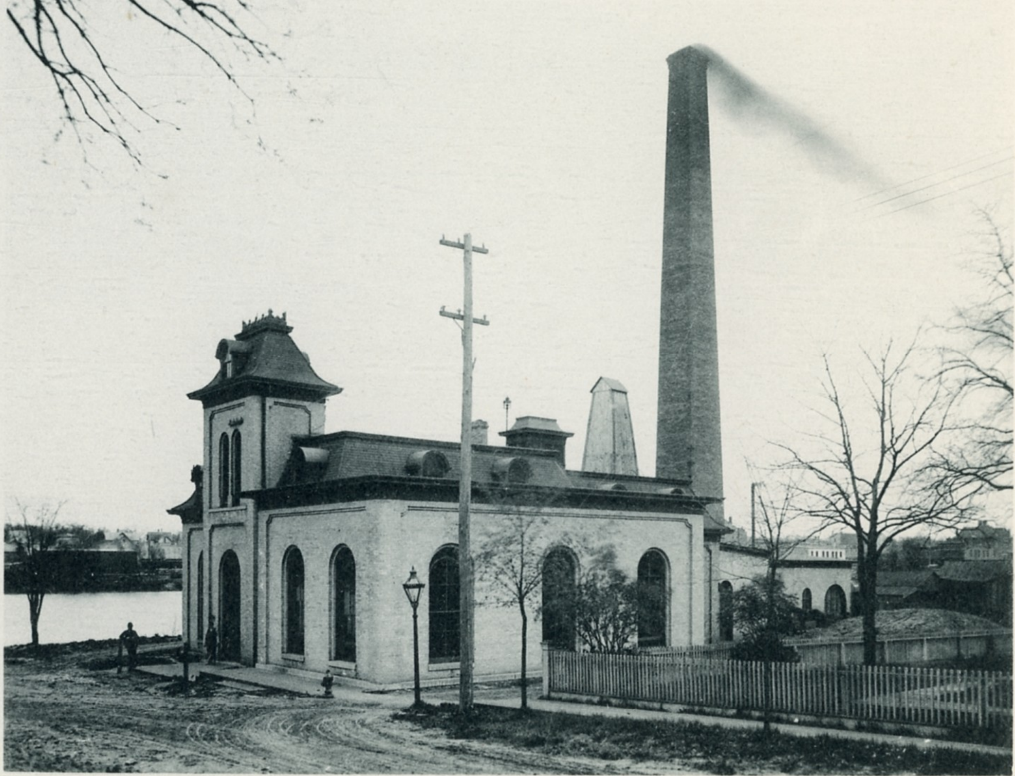
CITY WATER WORKS
