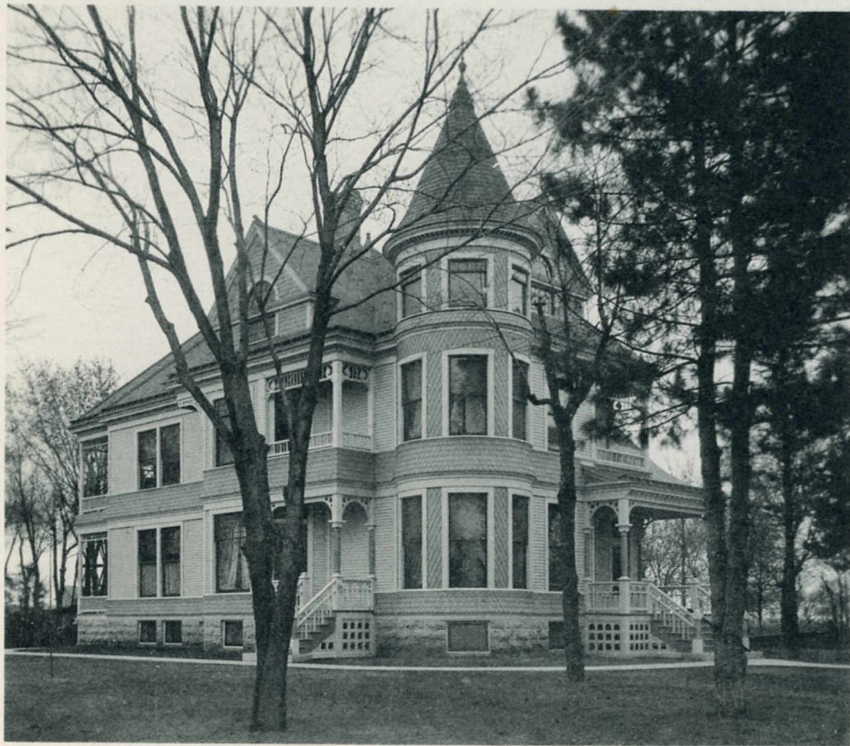
RESIDENCE OF HON. L. M. NOLING.
