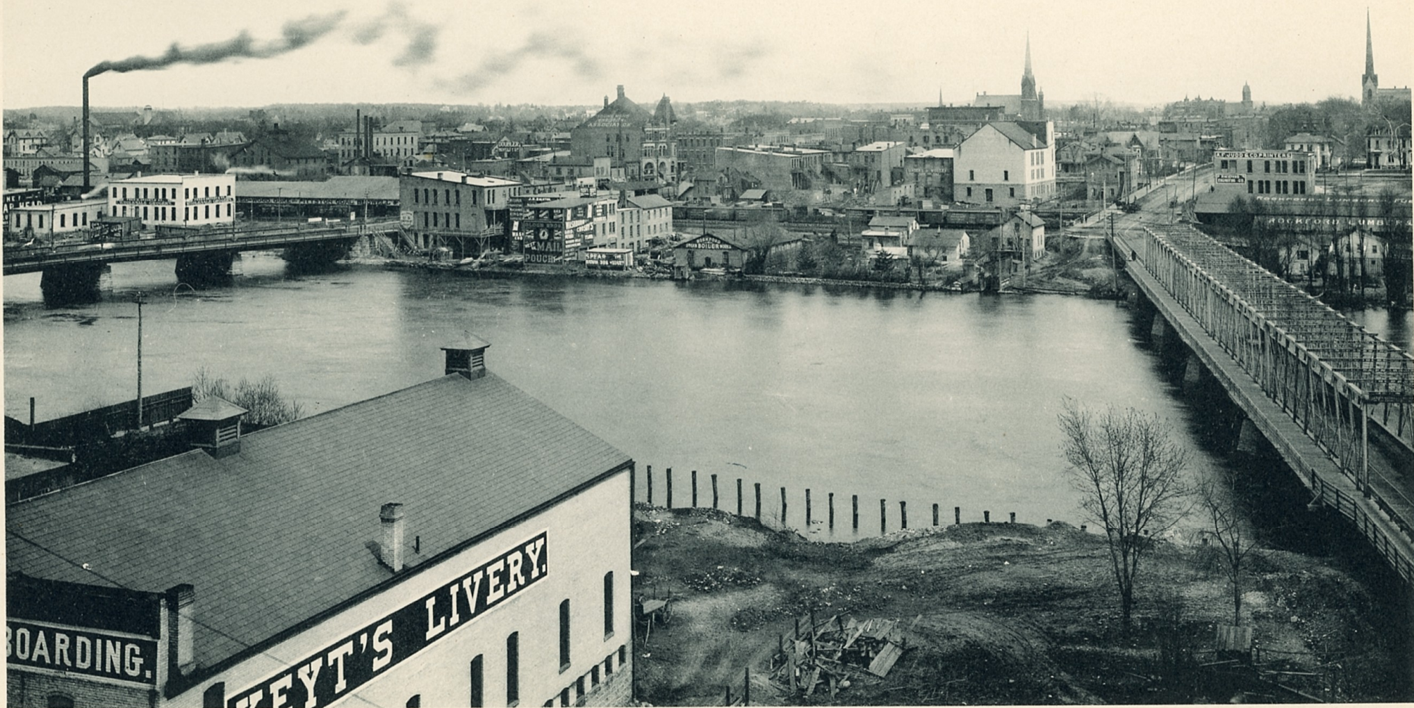
BIRDSEYE VIEW LOOKING EAST FROM WM. BROWN BUILDING.
